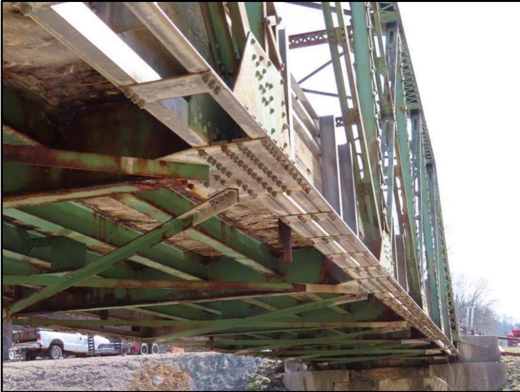
West/Downstream Truss, highlighting the Lower Chord arrangement. View SE, looking toward South Abutment (WVDOH 2-16-2022)
