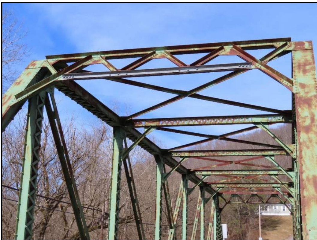
Highlighting Top of Bridge with Portal, Struts and Lateral Bracing. View NNW (WVDOH 2-16-2022)
