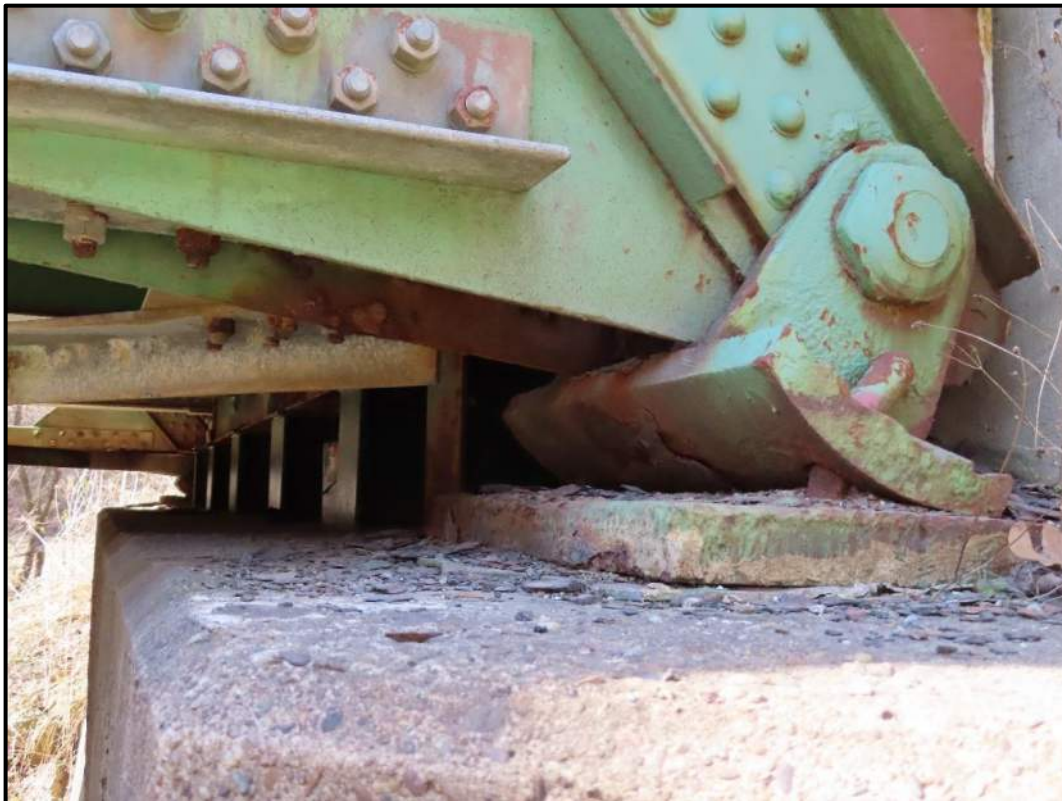
Rocker Bearing at South End Abutment. View E (2-16-2022)
