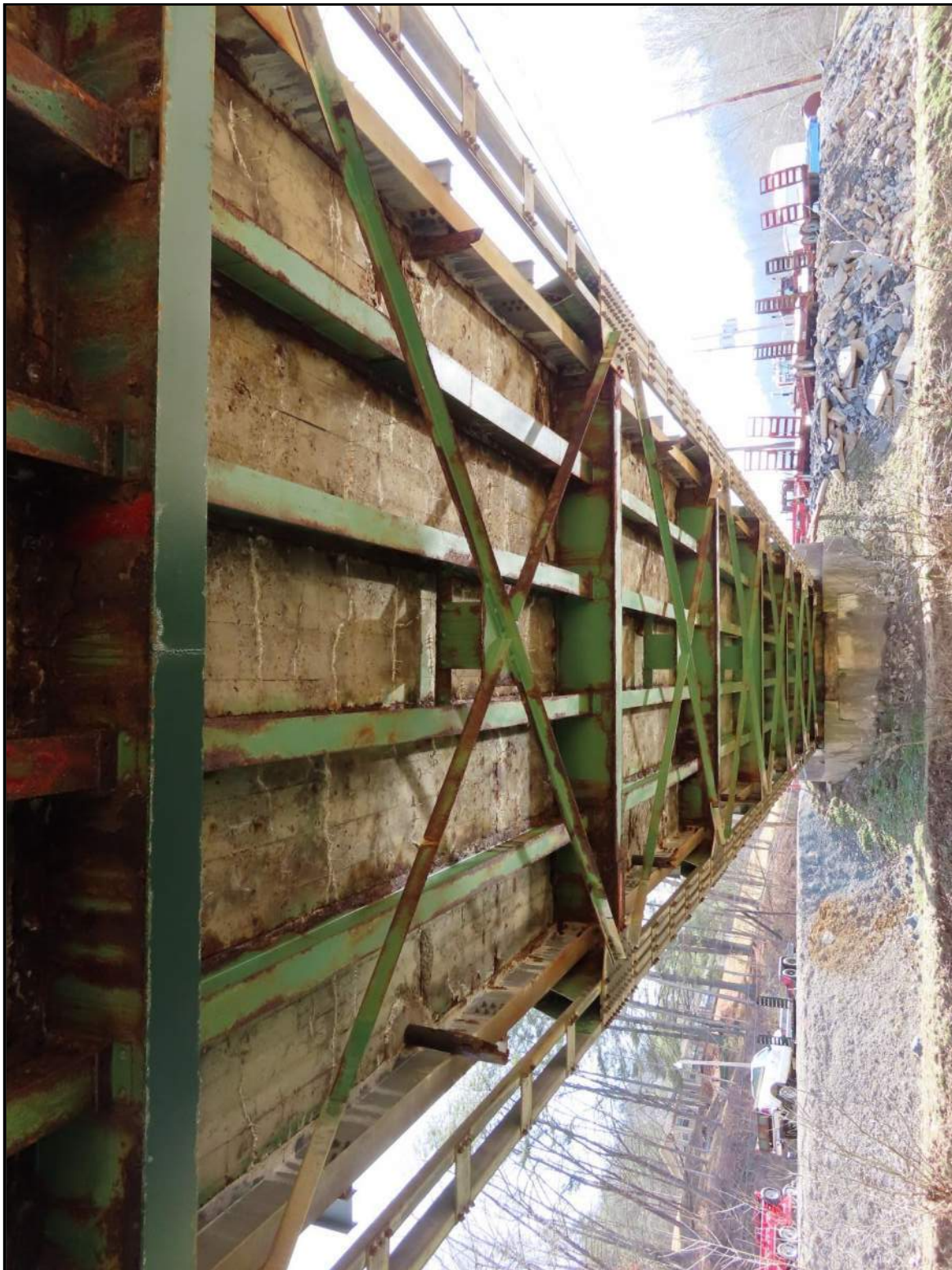
Underside of Superstructure, highlighting Floorbeams, Stingers and Lateral Bracing. View SE, looking toward South Abutment (WVDOH 2-16-2022)
