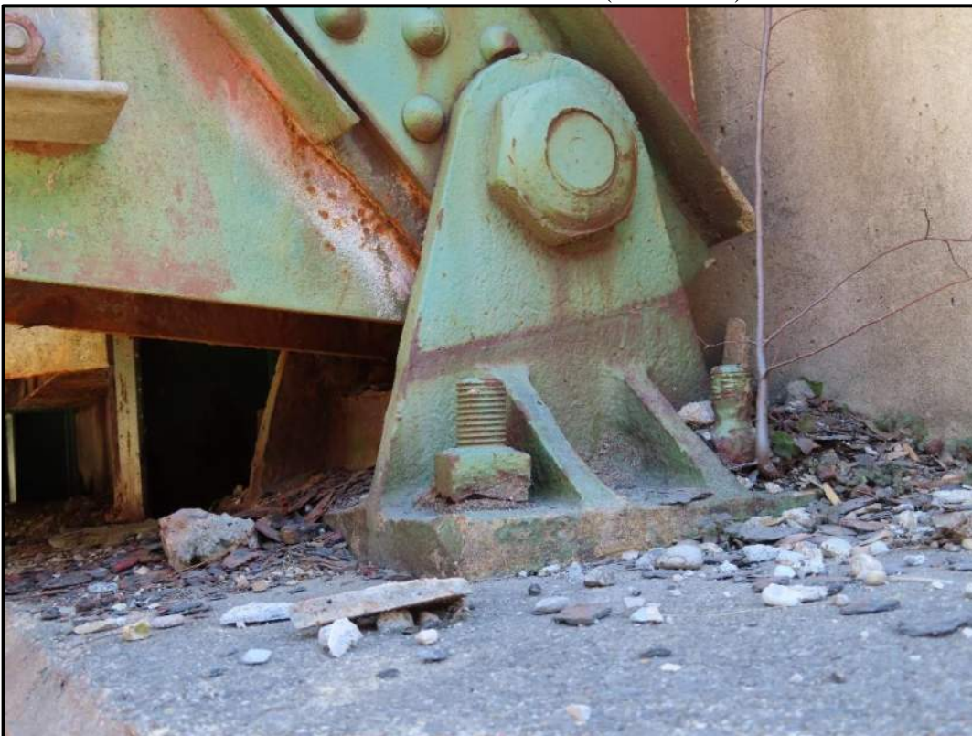
Fixed Bearing at North End Abutment. View W (2-16-2022)
