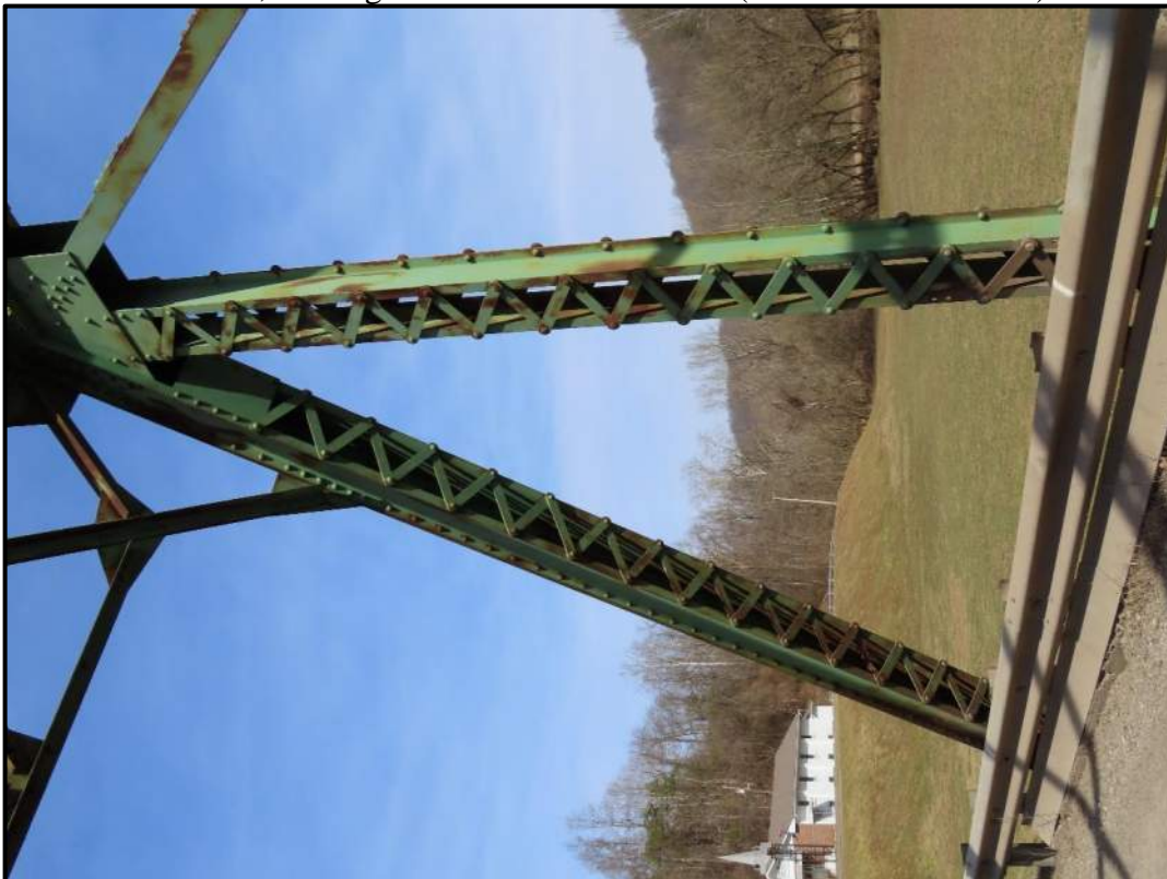
End Post and Vertical Post Details. View N (WVDOH 2-16-2022)
